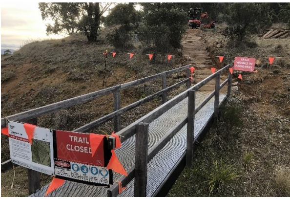
Work begins on the southern track Photo: Rob Lundie
